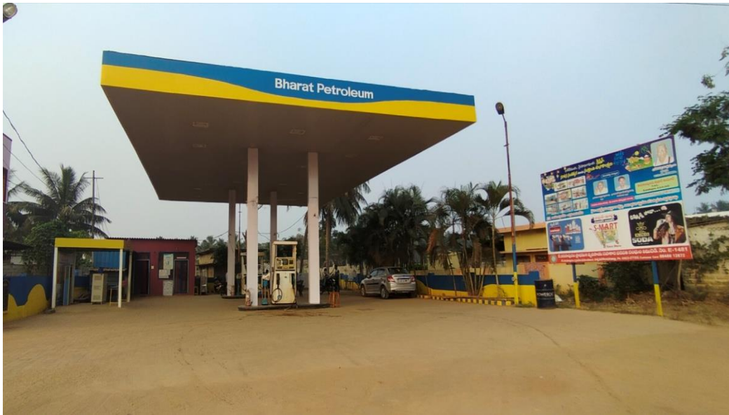
Fig. 10 Petrol and Diesel Pump
