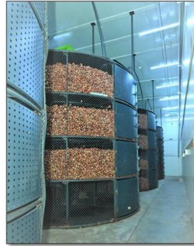
Fig. 8 Controlled Onion Storage Structure at Kala Biotech
