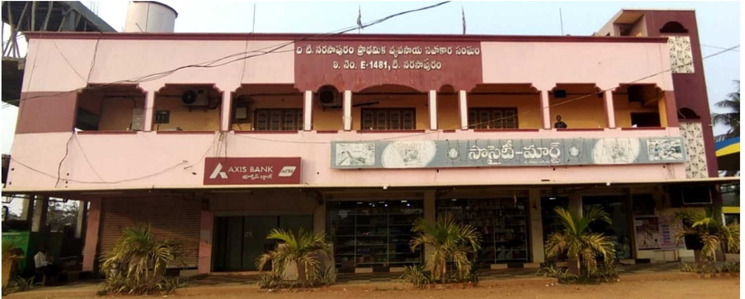
Fig. 2: T Narsapuram PACS Office Building
