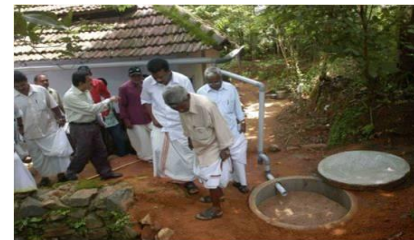
Fig 18 Dug-well Recharge
