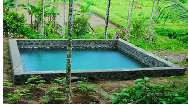
Fig 17 Embankment type pond
