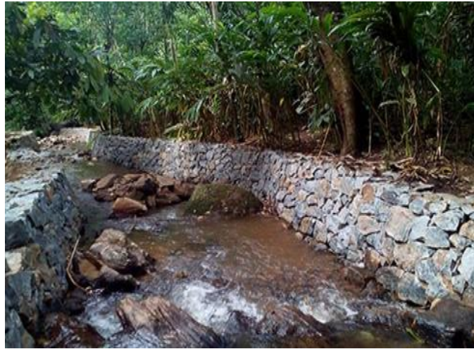
Fig 13 Stream Bank Stabilization
