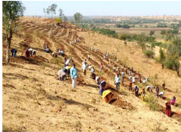
Fig 5 Contour trench
