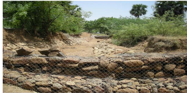
Fig 12 Gabion Structure
