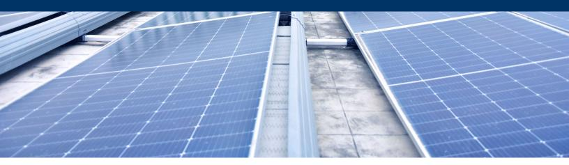
MANAGE installed 75 kWp Solar Rooftop Grid Connected system at the Academic Building, enhancing institutes self-sufficiency in power consumption to 75%.
