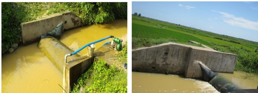
**Plate1. Rubber dams installed in watersheds of Odisha by IIWM, Bhubaneswar**
