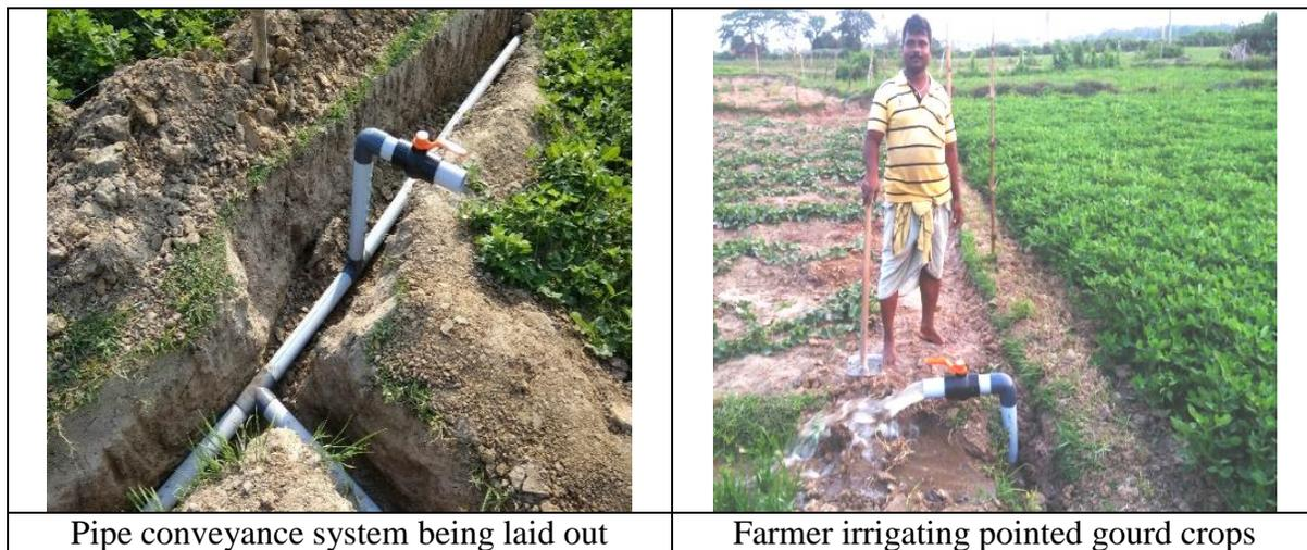
**(A) Dug well fed pipe conveyance based pressurized irrigation system (Ghurlijore minor irrigation system)**
