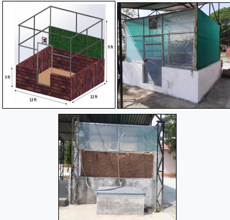
Fig.1: Evaporative cooling based hydroponic fodder production unit (Left: Design outline, Middle: Outside view- Front, Right: Rear side view)
