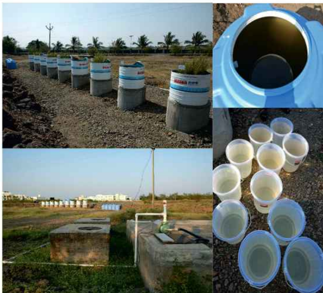
Fig.1 Pilot scale Subsurface-flow Constructed wetland system for treating wastewater generated from ICAR-NIASM, Baramati
