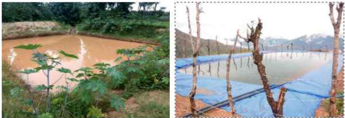
Fig. 5: Water harvesting structures: Poly-lined water pond for spring-water harvesting (left) and farm pond for rainwater harvesting (right).
