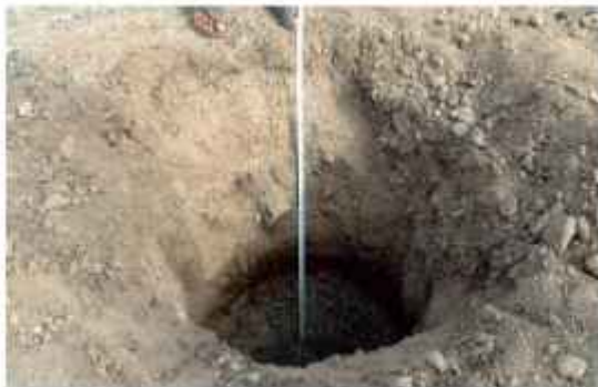
Depth of auger pit after blasting
