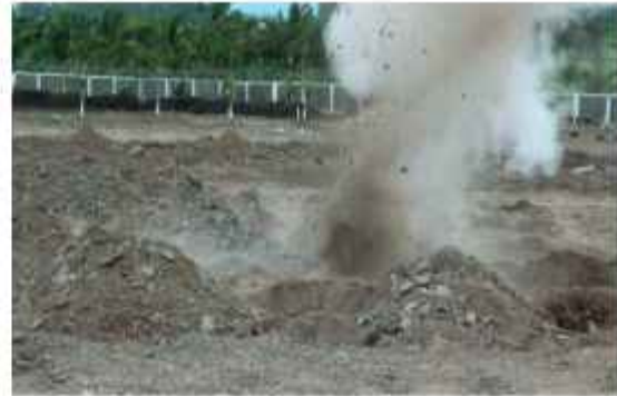
Micro blasting in pits
