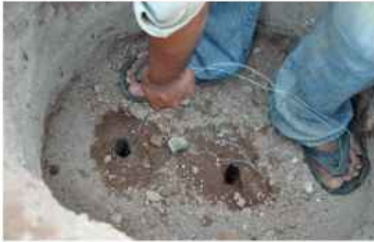
Inserting cartridges for microblast
