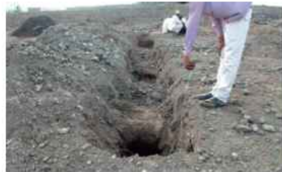
Depth of normal pit after blasting
