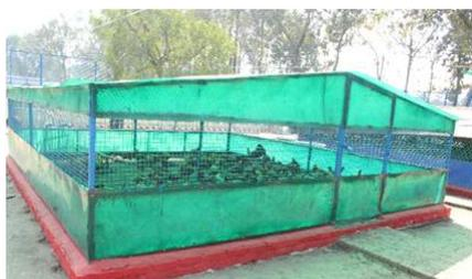
Fig. 4. Huts made of fiber sheet with square hollow iron pipe frame
