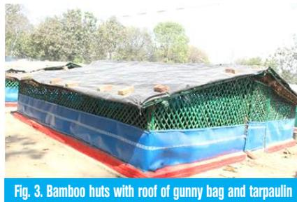
Fig. 3. Bamboo huts with roof of gunny bag and tarpaulin
