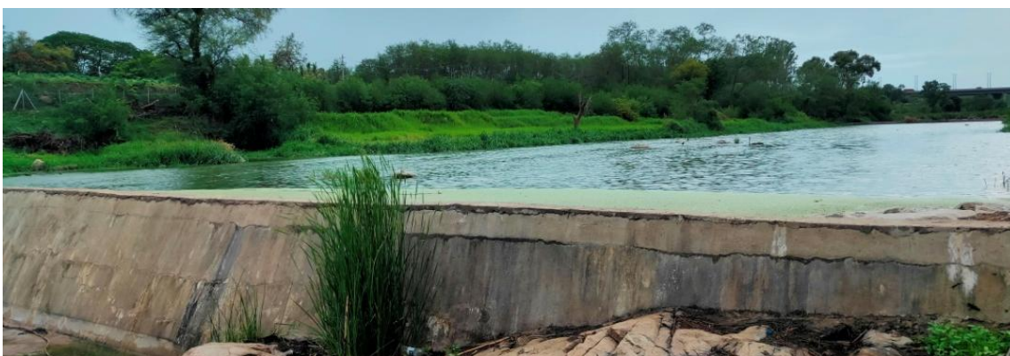
Water harvesting checkdam
