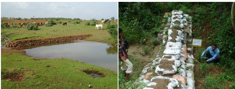
Earthen and bori bunds/sand bag checkdams
