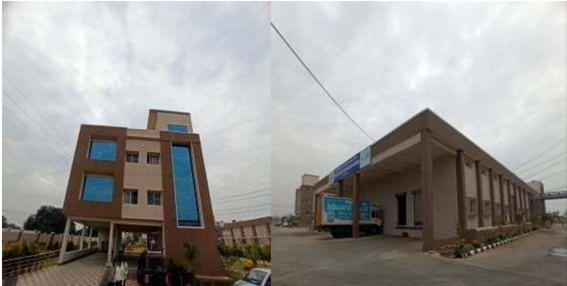
Fig.11: Administration Block in the new dairy farm.
